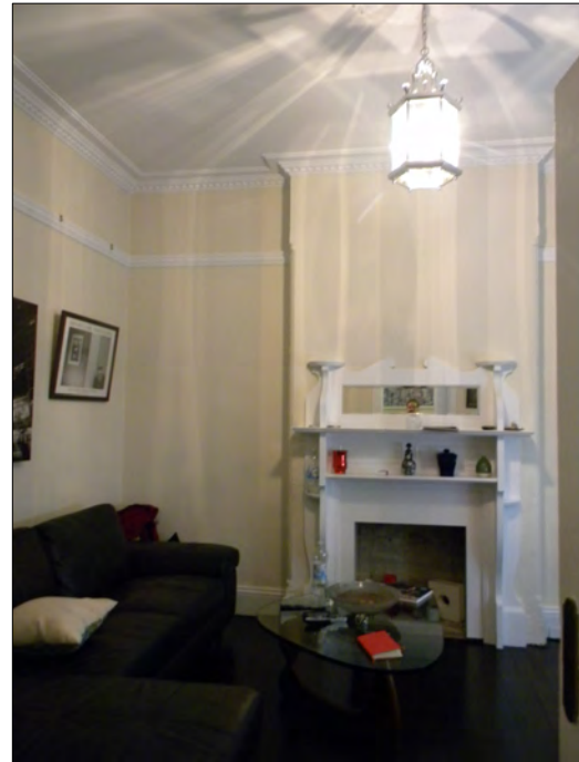
Figure 12: Fireplace in the front room at ground floor level, also showing ceiling and cornicing and picture rail.
