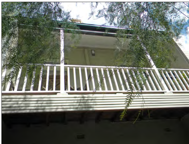
Figure 8: Detail of the first floor verandah.
