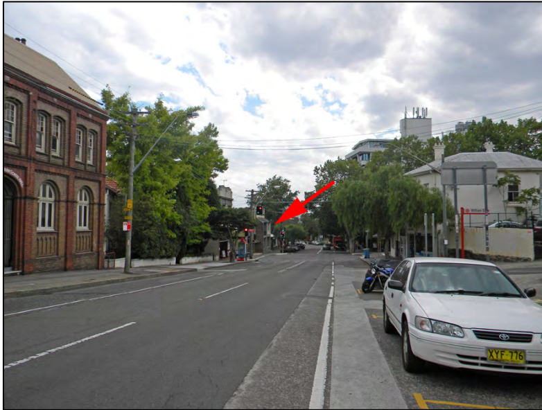
Figure 38: View south along Blues Point Road towards the site.
