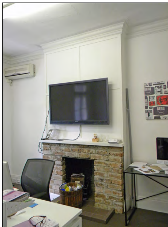
Figure 35: Fireplace in the front room, also showing skirting board profile, picture rail and cornice.
