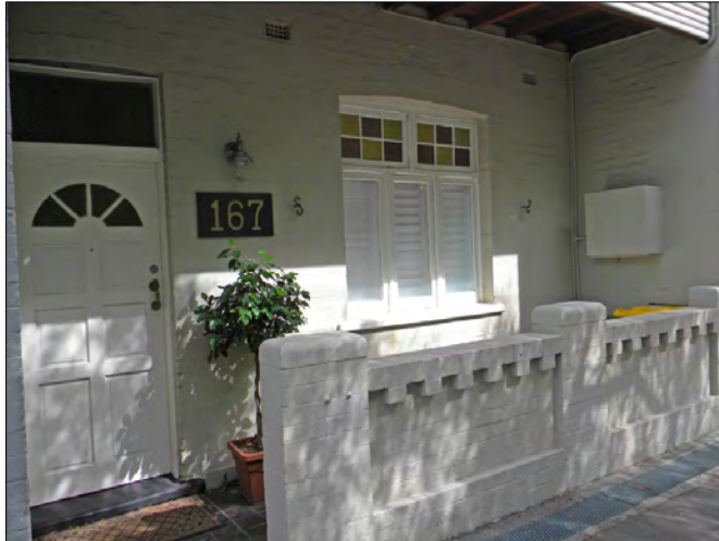
Figure 7: Ground floor verandah and front elevation. Note the shutter clips, indicating that this window may have once had shutters.
