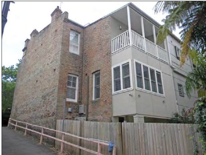
Figure 9: Southern and eastern elevations of the principal building form and the rear wing.
