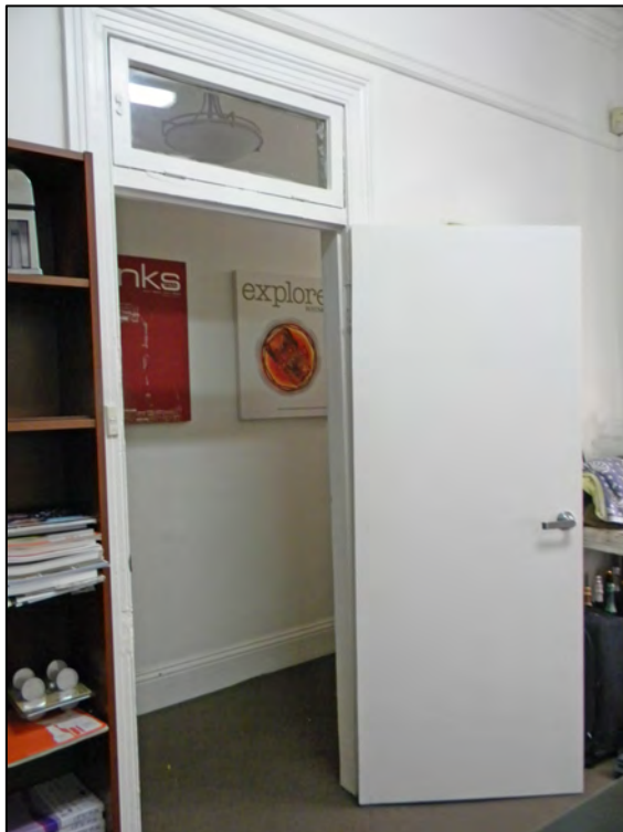
Figure 28: Typical door, ground floor.
