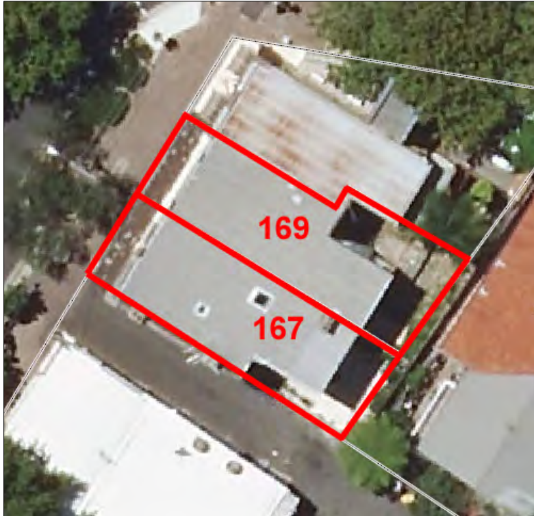
Figure 4: Aerial photograph over the site. SIXMaps.
